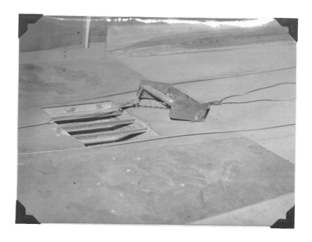
Figure 3. Photograph of Box Type Scraper with the blade bolted at a 30 degree angle to the line of pull.
