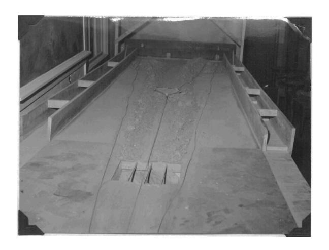
Figure 6. Photograph of Slope Bail Hoe Type Scraper moving mixed-size rock. Note ridges built up along path of scraper.
