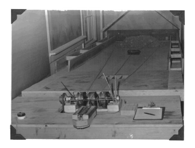
Figure 5. Photograph showing electric hoist assembly and table.
