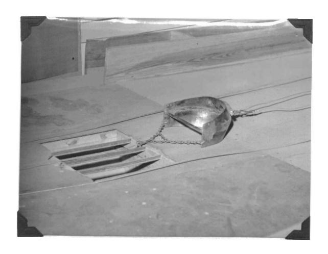
Figure 4. Photograph of a Crescent Type Scraper. This model has a digging angle of 60 degrees.
