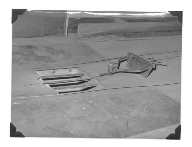
Figure 1. Photograph of Straight Bail Hoe Type Scraper with the blade bolted at a 45 degree angle to the line of pull. Note counterweights on bail and baffle plate.
